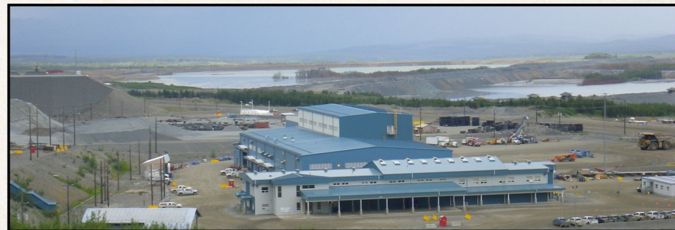
Mt. Milligan concentrator, tailings ponds in background
