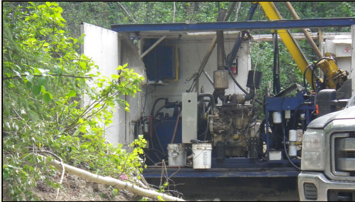
Drill rig at Snowbird
